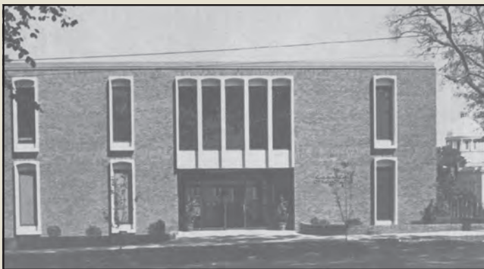
New League Headquarters at 535 Adams Avenue, 1970. The Capitol can be seen at right.
